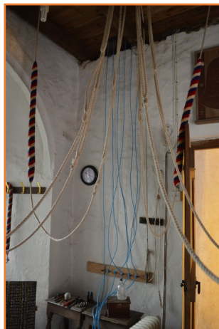
Installing the new (blue) ropes
